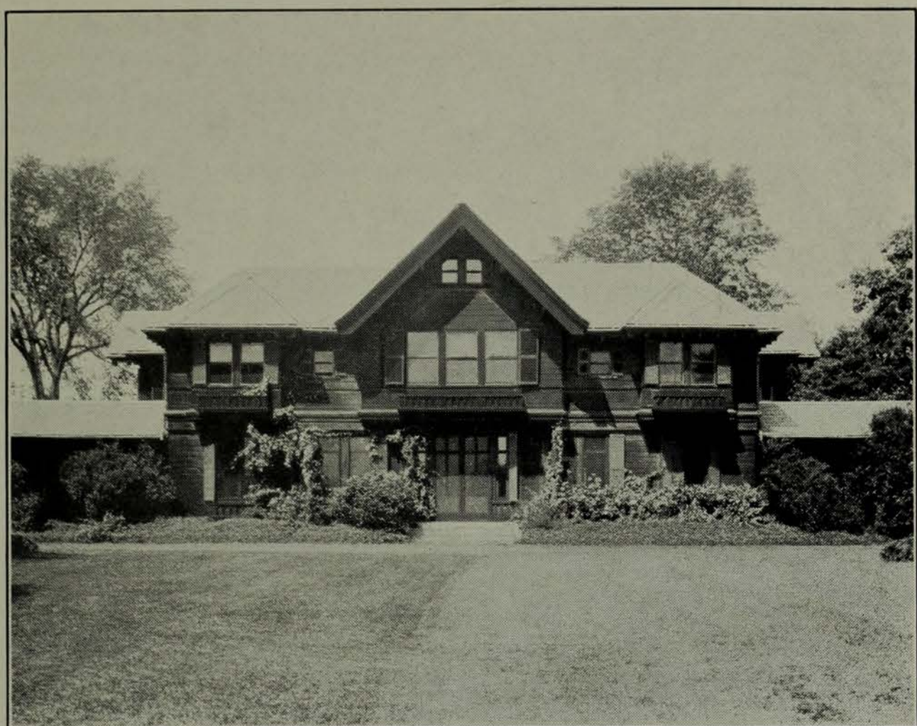
THE GUEST HOUSE, SOUTH FRONT
