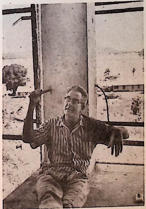
■ Metalanim Bay behind him and a moment's rest to plan the unfinished school.
