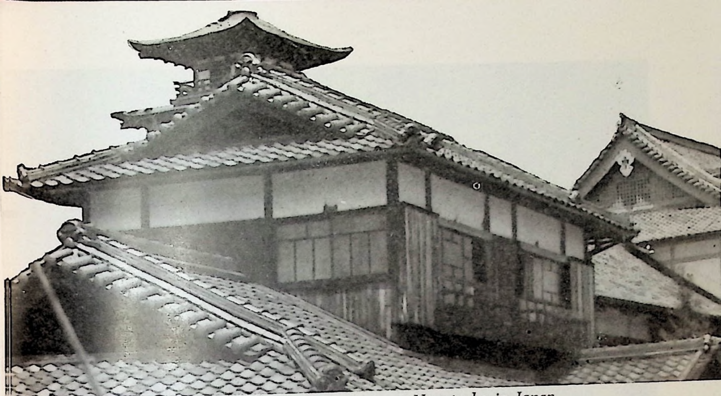
The typical Buddhist roof of the Jesuit Novitiate at Nagatsuka in Japan.
