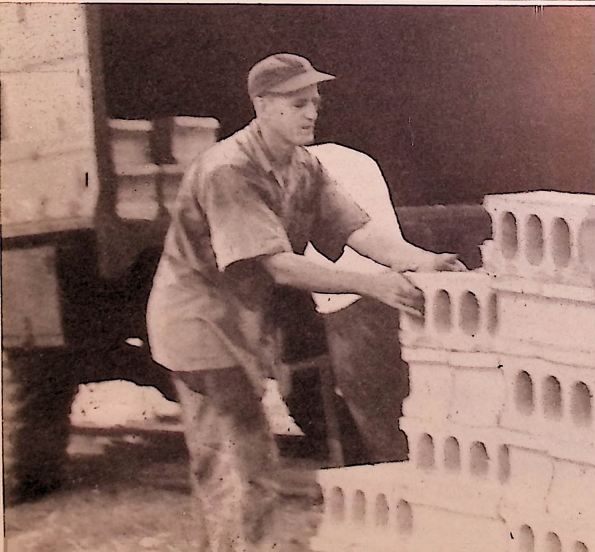
Father Lange loads cement blocks for new Trincomalee sch.
