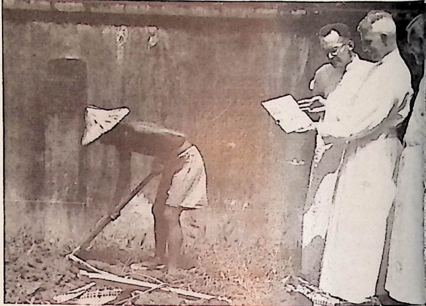
Inspecting building permit on site of new library for Catholic. Monsignor Eugene Fahy S.J., Prefect Apostolic of Yangchun; Father Paul O'Brien S.J., Mission Superior; Father Murphy S.J., Mission Superior.
