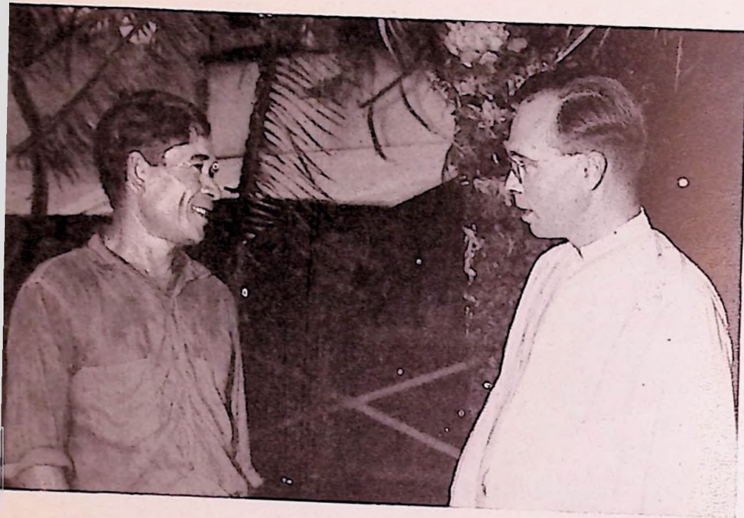
Edwin Capelle, Likiep's comedian and also one of its best carpenters, chats with Father Donohoe about the latter's job of rebuilding on Jabwor island.
