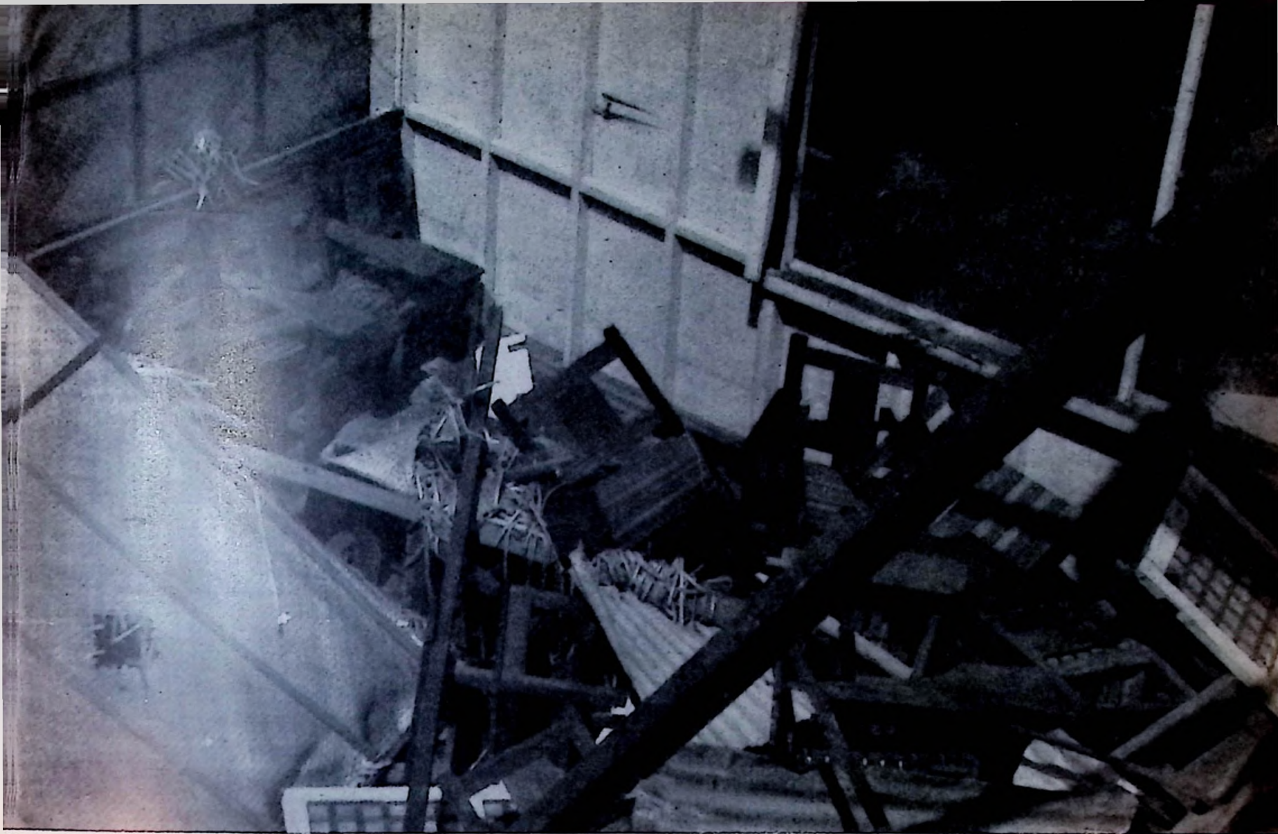
This is one of the rooms at Naga after the typhoon.
