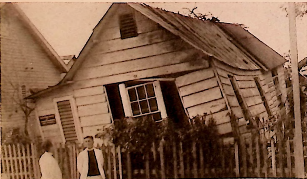
Fathers Edmund Cheney, S.J., and Joseph Dooley, S.J., inspect the damage after the recent hurricane in Jamaica.
