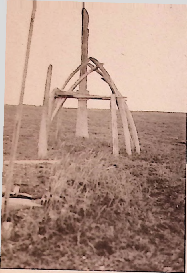
(Left) The first steps in the making of an Eskimo hut, setting the whale bones in place. (Above) An ancient cemetery; bones again served a useful purpose.
