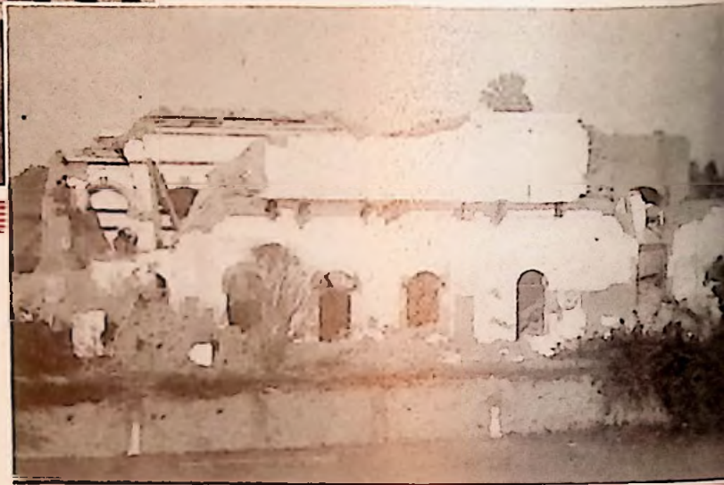
After the earthquake.
