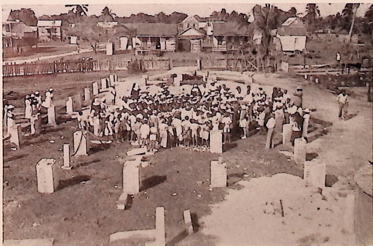
(Below) Stann Creek gathers to mingle its tears with ashes of 75 years.
