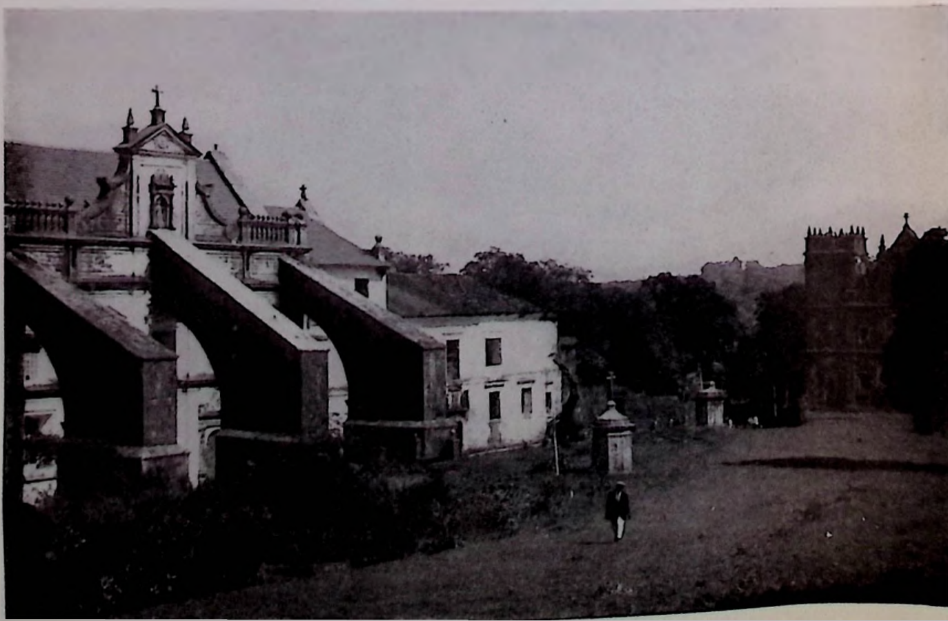
The flying buttresses of St. John's Church, Goa.
