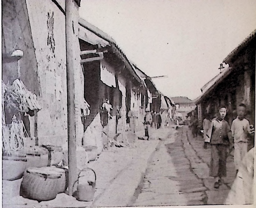
A typical street in Shuyang. Many of these houses were destroyed by fire and shells.
