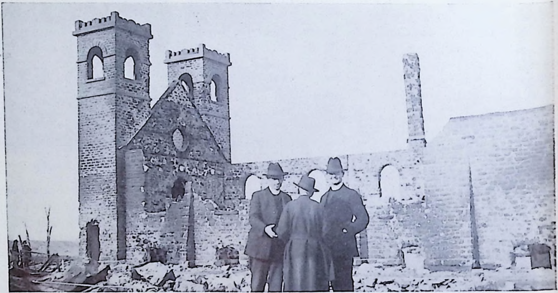
Father Walter Fitzgerald, S.J., (right), newly appointed Coadjutor Bishop of Alaska is no stranger in the mission field. He is shown here with Father Balfe, S.J., and Father Feusi, inspecting the ruins of the church at St. Paul's Indian Mission, Montana.
