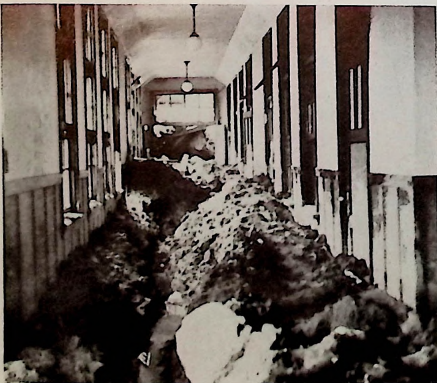
Stones and boulders choked the corridors.
