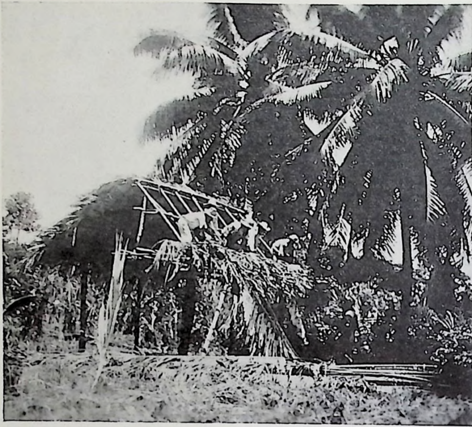
A thatch-roof house in the making at El Cayo.
