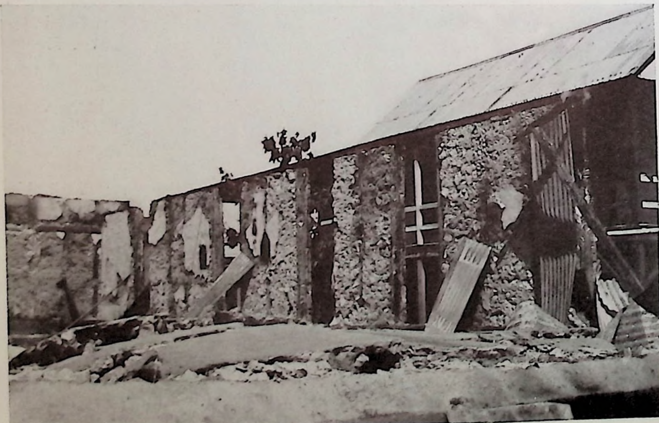
The house of the Padre is just outside the ruins of the church. Fortunately there was no wind the night of the fire, for if there had been, the house, too, would have been destroyed.
