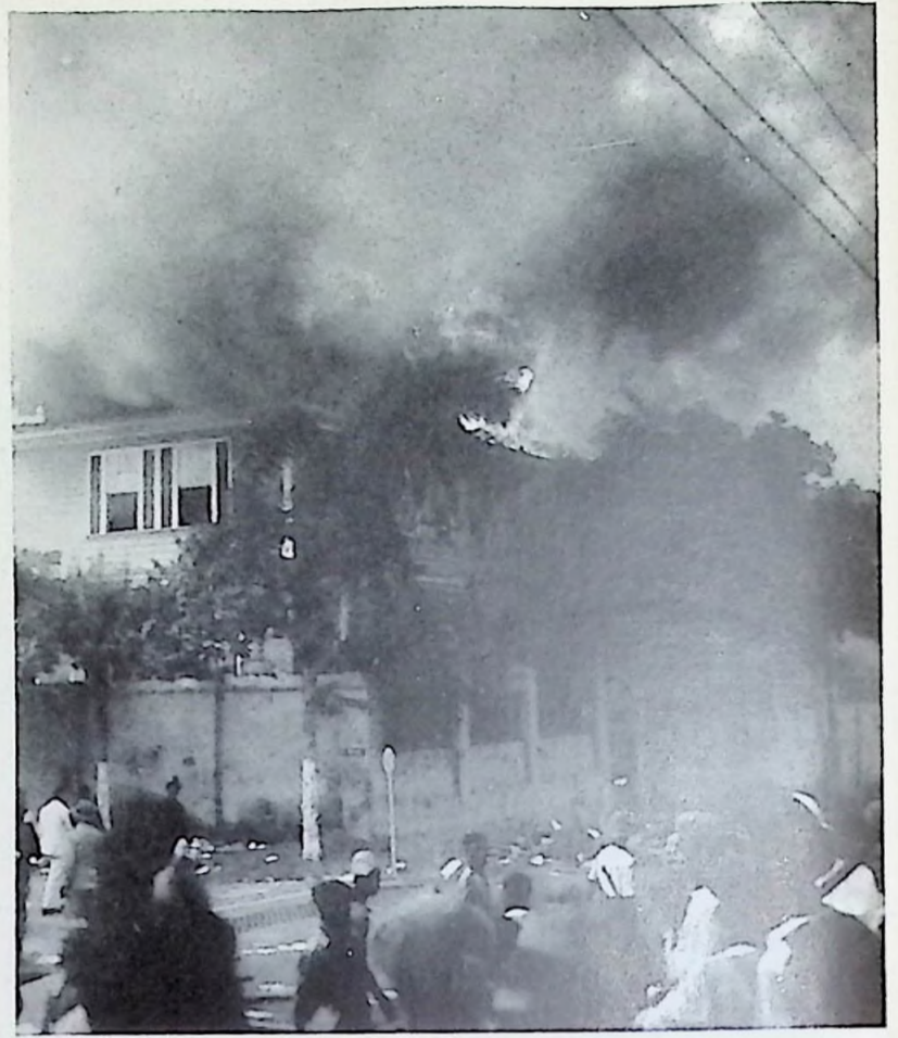
The northwest corner of the Immaculate Conception High School at the height of the fire.
