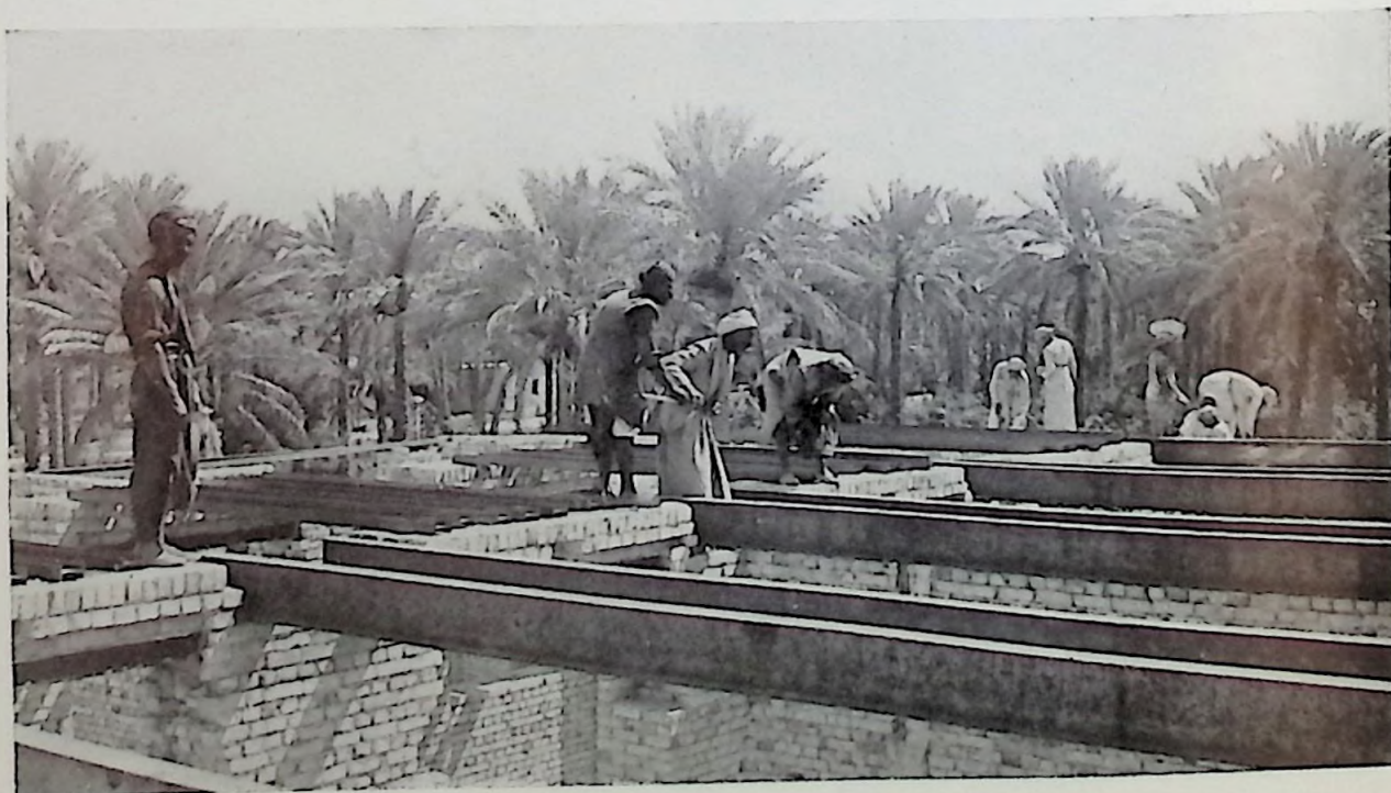
Going up. Baghdad College rises brick by brick. Incidentally, each beam is raised from the ground by sheer muscle and brawn. Mechanical aids are not used.
