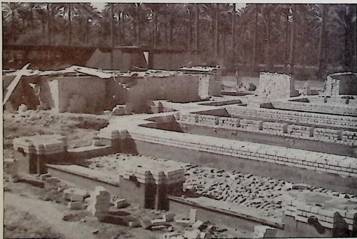
Construction work for the new building of Baghdad College, Baghdad, Iraq.
