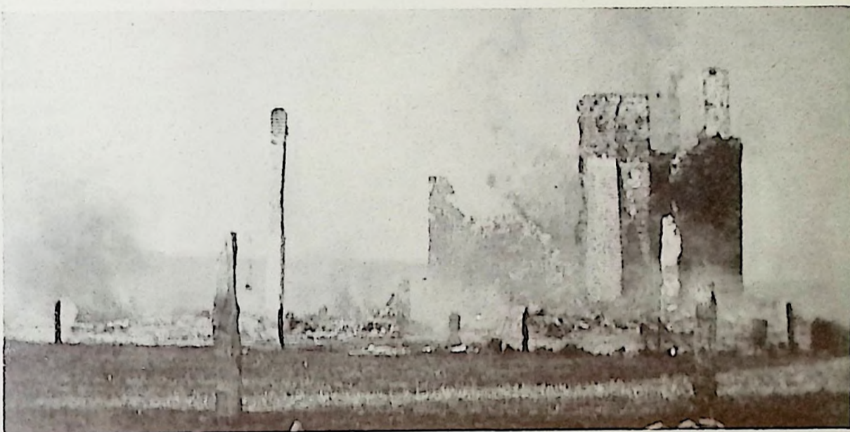
Early in November, 1931, a fire, starting in a defective flue, destroyed nearly all the buildings of St. Paul's Mission, Blaine Co., Montana. Nothing was left except the boys' building, which also housed the dining hall, post office and administration office.
