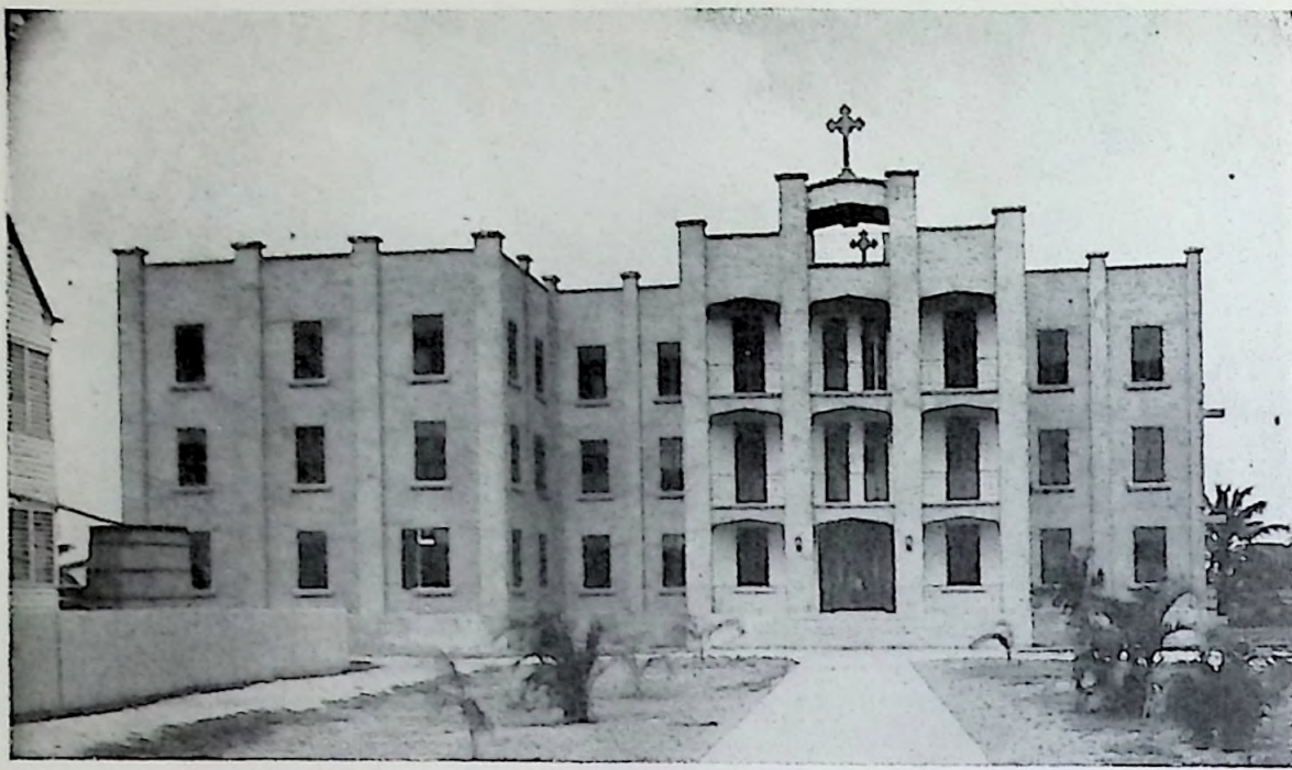
New reinforced concrete convent and school of the Sisters of Mercy in Belize. It was built under the direction of Very Rev. Martin M. O'Connor, S.J., Superior of the Jesuit Mission of British Honduras.
