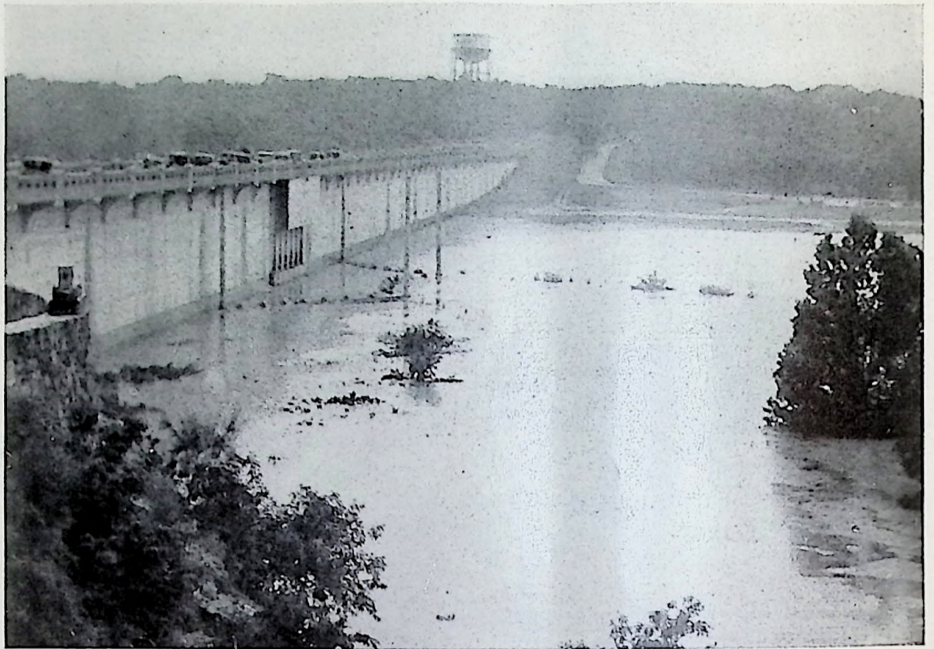
The San Antonio emergency dam as it appears after a Texas storm.
