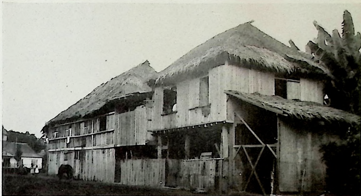
Where Father Consunji, S.J., stakes his claim. The only permanent Catholic rectory from Aparri to Jolo, which is constructed merely of nipa material.
