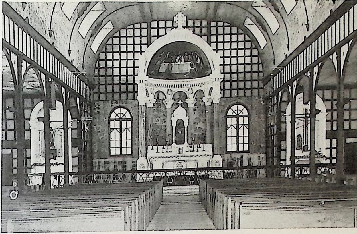
Interior of new church, showing the altar done in cement from a model generously supplied by the Frederick Pustet Company.
