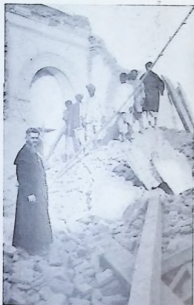
Bishop Bernard J. Sullivan, S.J., at Bettiah, inspects what is left of the largest parish church of his diocese. It required two days of digging to rescue the Blessed Sacrament from these ruins and raise it again on high.
