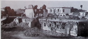
At Bettiah, the Knitting School (white building in the rear) was badly damaged interiorly. The wreckage in the foreground is all that is left of the missionaries' residence.
