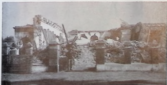
The Church of Chhabari after the earthquake. It took three days to recover the Blessed Sacrament, and when the Tabernacle was finally uncovered it was a marvel to see that in spite of the mass of bricks, pieces of concrete and heavy iron girders that were piled all around, the tabernacle was scarcely scratched. From this abiding Presence of their God comes inspiration for reconstruction.
