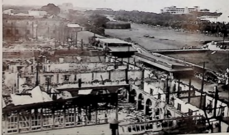
The ruins that tell the sad story of the destruction by fire, August 13, 1932, of the Ateneo de Manila, the famous college of the American Jesuits of the Maryland-New York Province in Manila, P. I.
