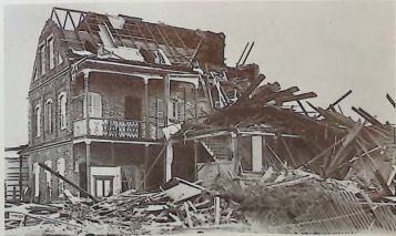
All that the hurricane left of five buildings of the Sisters of Mercy.
