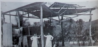
A dilapidated barrio church—one of the 24 stations in Lanao—where Father Hofmann says Mass. Father Hofmann (left) and the author.
