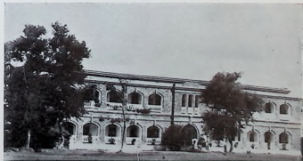
The new dormitory building at Khris Raja High School , Bettiah, Patna Mission, is the gift of an Indian ruler, the Bettiah Raj .
