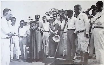
Very Reverend Charles H. Correa, S.J., Prefect Apostolic of the Magdalena River Mission, blessing the beginning of construction on a new road in his territory.
