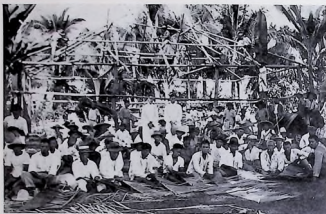
Preparing to put the dispensary under its nipa roof.
