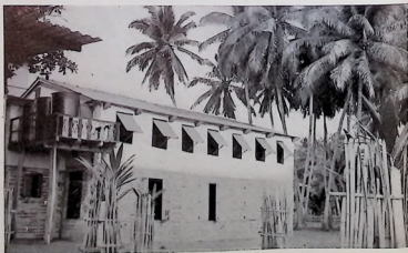
"The first story he erected in concrete . . . The second story is of wood."
