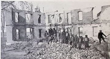
"The school and mission church were reduced to ruins."
