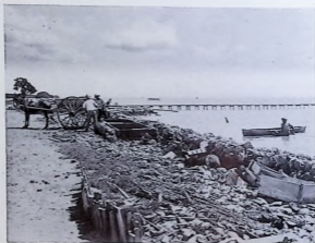
Working against odds, building a protecting sea-wall.
