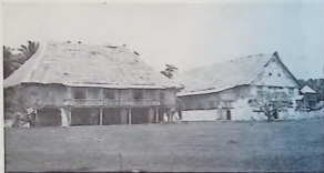
Convento and Church at Oroquieta.
