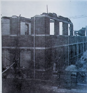
Tokyo University after the earthquake
